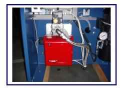
When there is a modulating burner (BS3/M) installed, the lowest possible power output must be regulated below 60kW !!!
